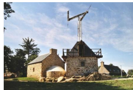
Station Chappe de Saint-Marcen.
